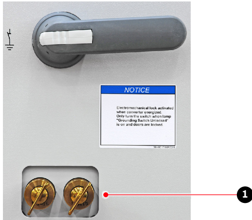
Figure 12 – Example of a customer-specific trapped (1) key interlock system
